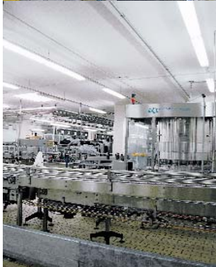
◀ Post-installation lighting for the production area
